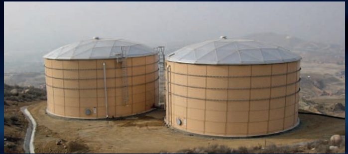
▲ Multiple potable ground storage tank facility.
