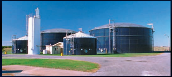
▲ Sludge stabilization and sludge storage facility.
